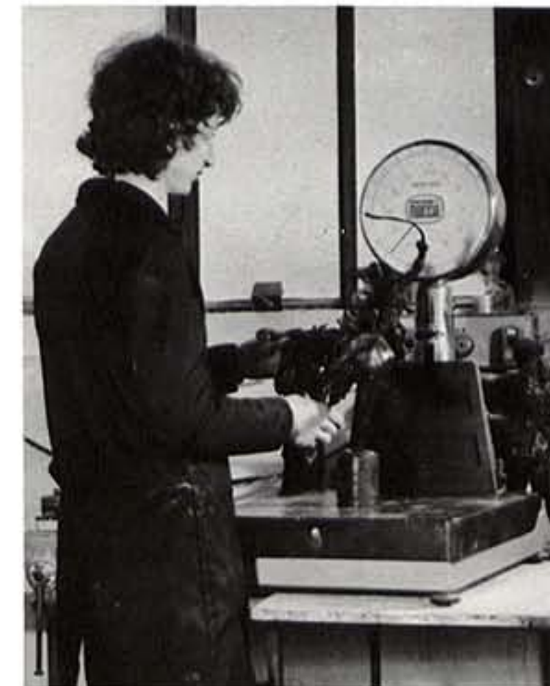
5. Ivano Bigicchi measuring the exact weight of a finished casting
